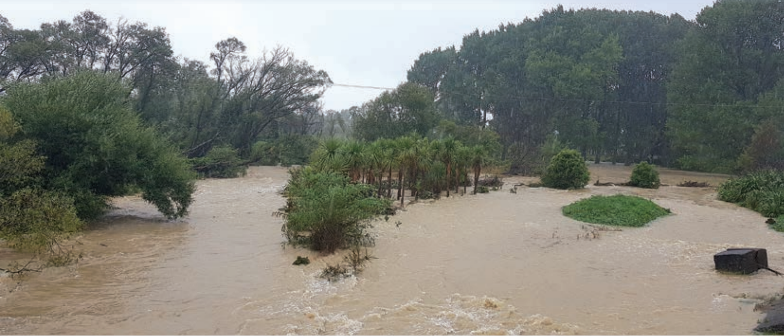
View looking north off Belvedere bridge in the floods last year
