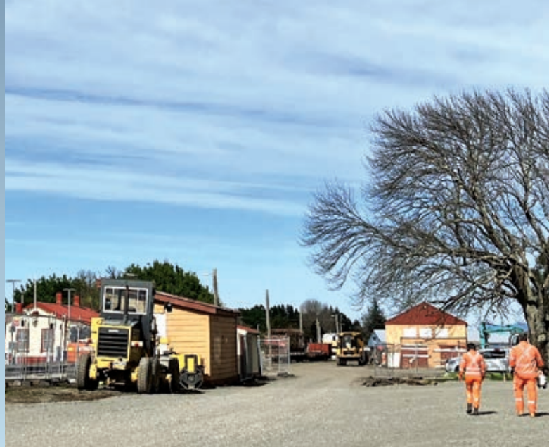
KiwiRail has prepared the site
