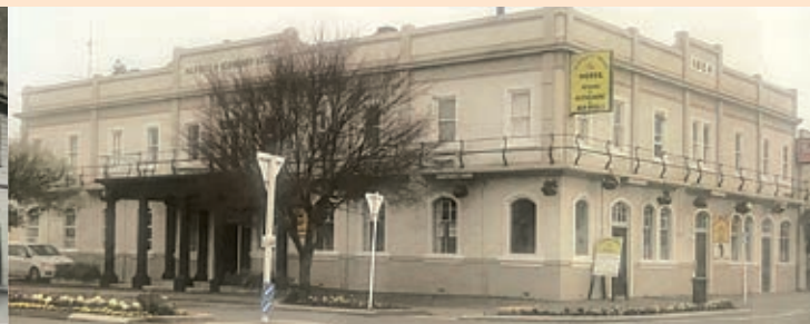
The original wooden structure, and the concrete replacement of 1924
